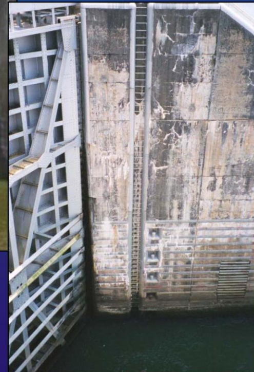
Concrete deterioration at Chickamauga
