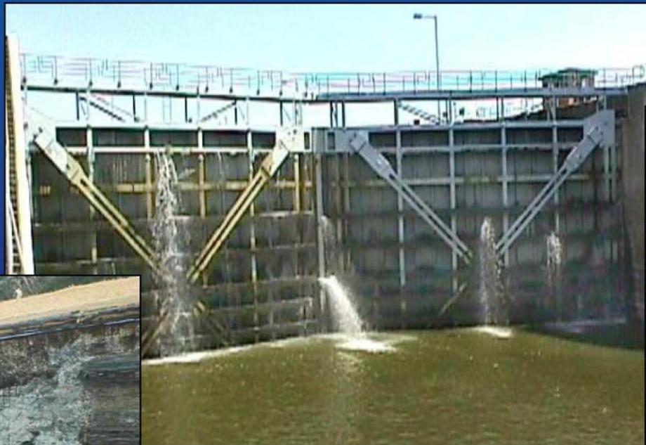
Leaking miter gates, Upper Miss Lock 19
